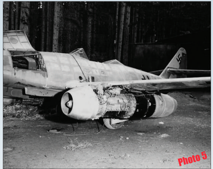
▲ The Me 262B fuselage differs considerably from the single-seat version, with a much-lengthened cockpit and raised fairing ahead of the tail for the canopy.
